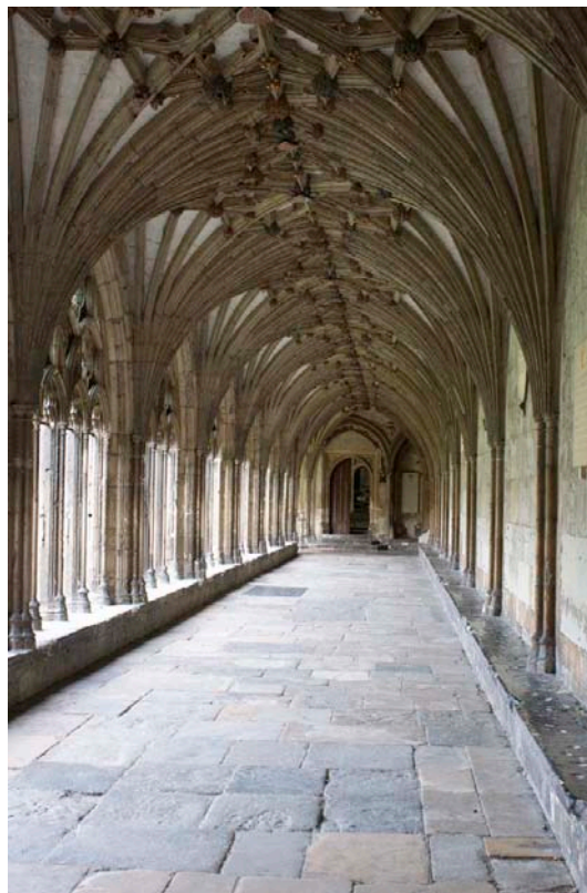
Canterbury Cathedral cloisters
